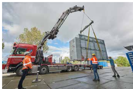
PYRENA-PYPO pilot plant arriveert op de Green Chemistry Campus
